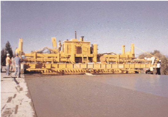
Figure 3-1. Fly ash improves workability for pavement concrete.
